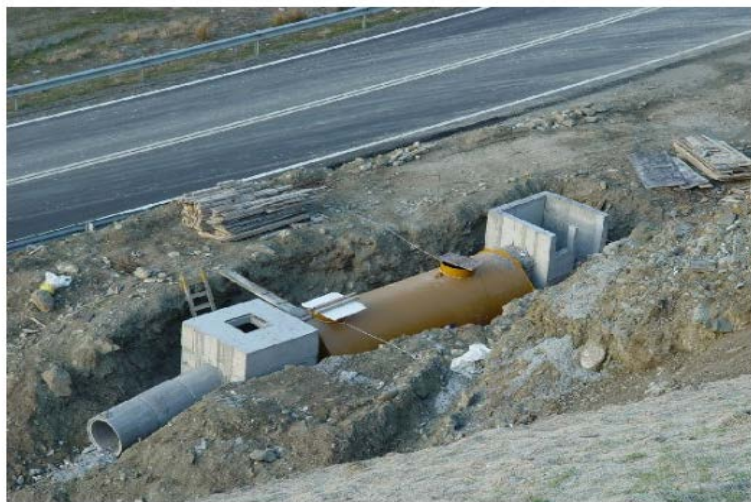
Photograph 3. Pollution Contro Unit under construction
